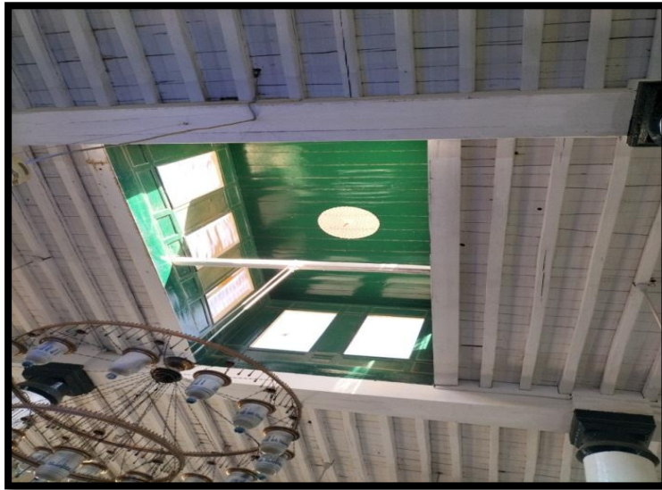
(Pl. 17) The Skylight in the middle of the mosque's Ceiling.
